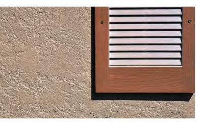
Cementous stucco is a porous material that is commonly used to finish the exterior of new homes. Minor cracking (also known as "hairline cracks") may appear in the topcoat of the stucco over time – this is normal and will be most noticeable on smooth finish coats.
